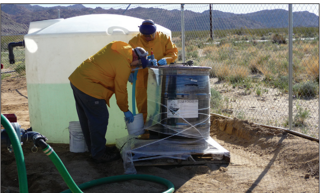
Left: The regeneration team and researchers collect water samples from tank B during the regeneration process. Right: Regeneration team members prepare the caustic regeneration solution in the storage tank.
