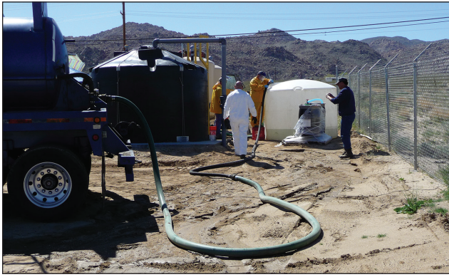
Left: Regeneration team members pump the caustic solution to the tanker for disposal. Right: A tanker truck is used to haul wastewater to an industrial chemical disposal facility.
